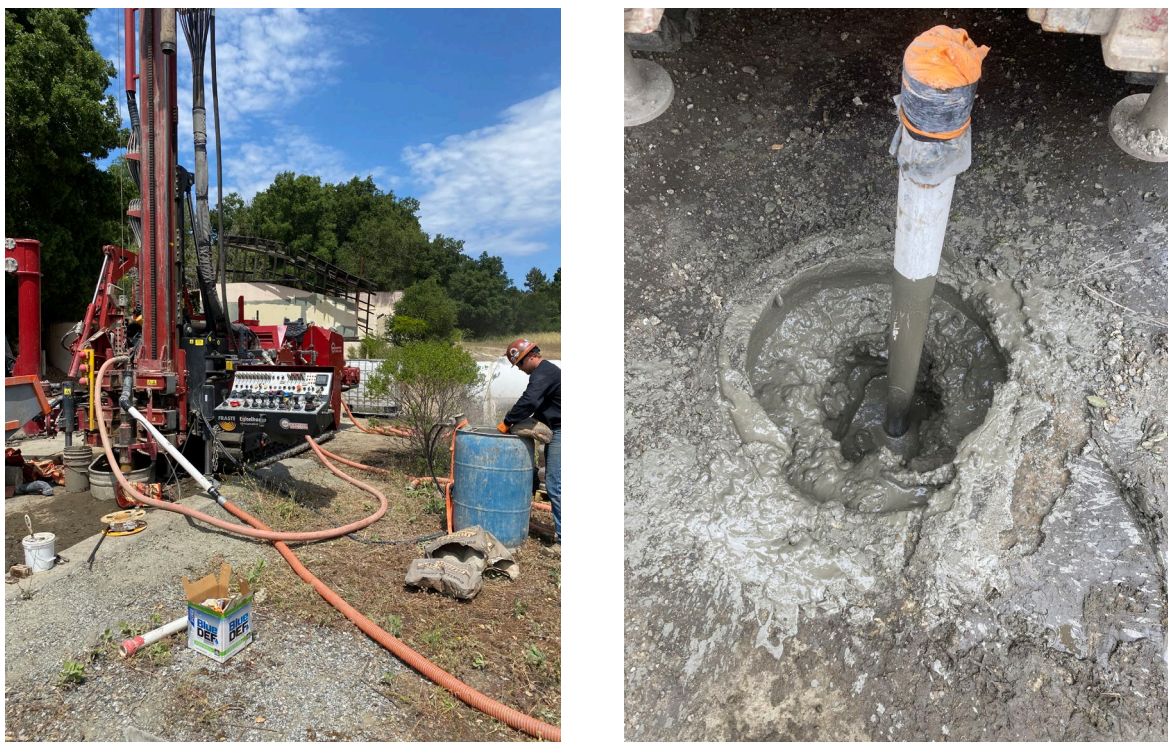
Figure 9. Example Annular Seal Placement
