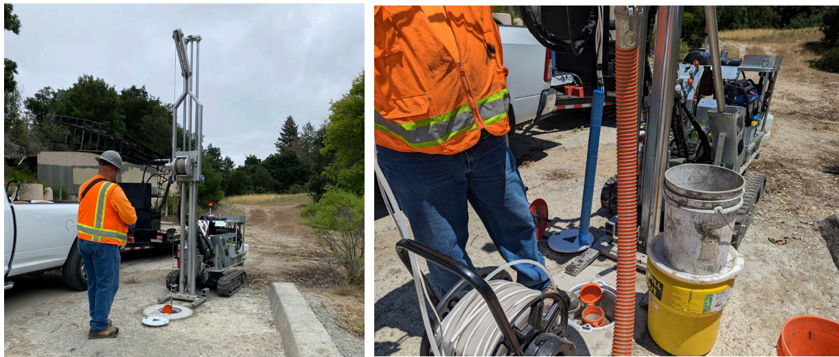
Figure 11. Well Development Rig (left) and Submersible Pump (right)
