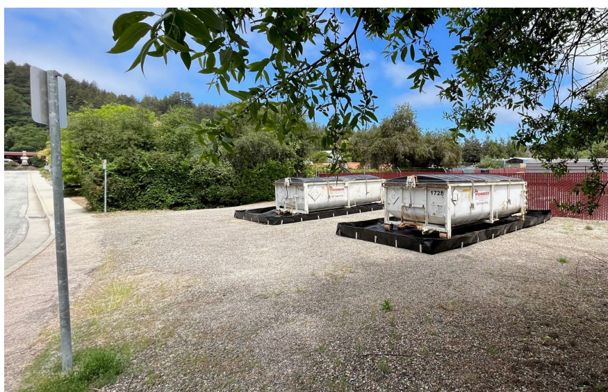
Figure 12. Roll-off Dumpsters and Secondary Containment
